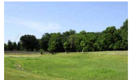
Example of a dry detention basin
