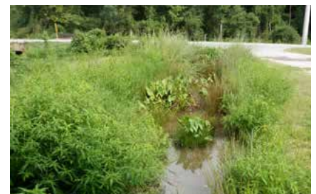
Example of a green route swale
