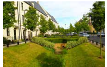
Example of a road side swale
