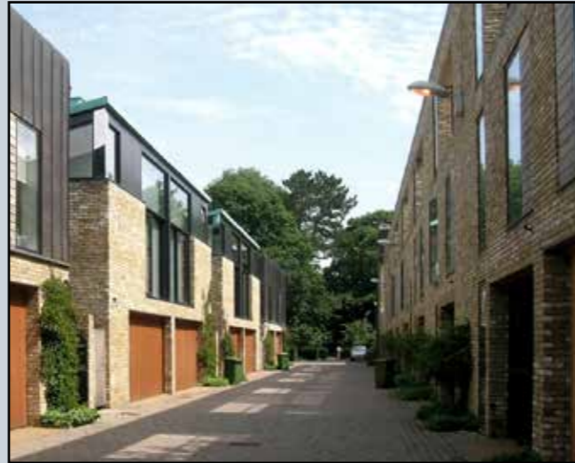
High Density - @ 55dph Contemporary A combination of apartments and Mews houses with on plot integral parking
