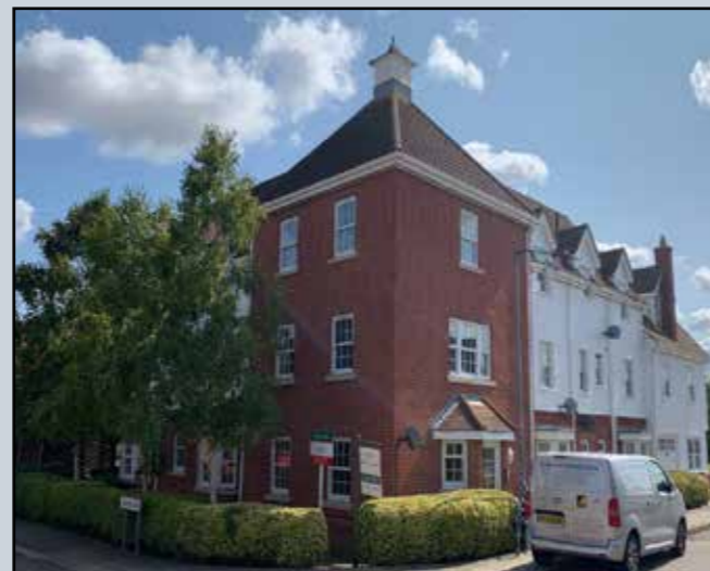
High Density - @ 55dph Traditional A combination of apartments and houses with rear courtyard parking
