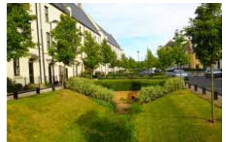
Example of a road side swale
