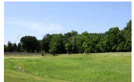
Example of a dry detention basin
