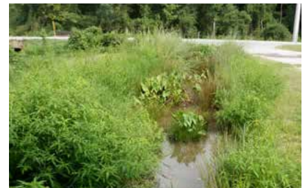
Example of a green route swale
