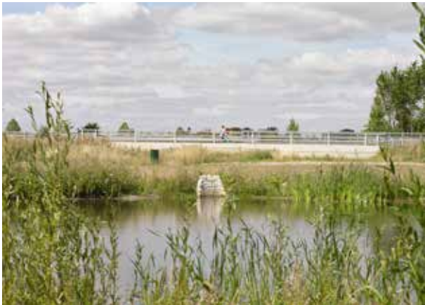
Example of a permanently wet pond
