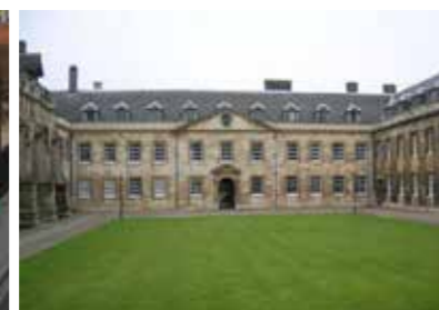
Fig. 86: Example of Grand Court entrance
